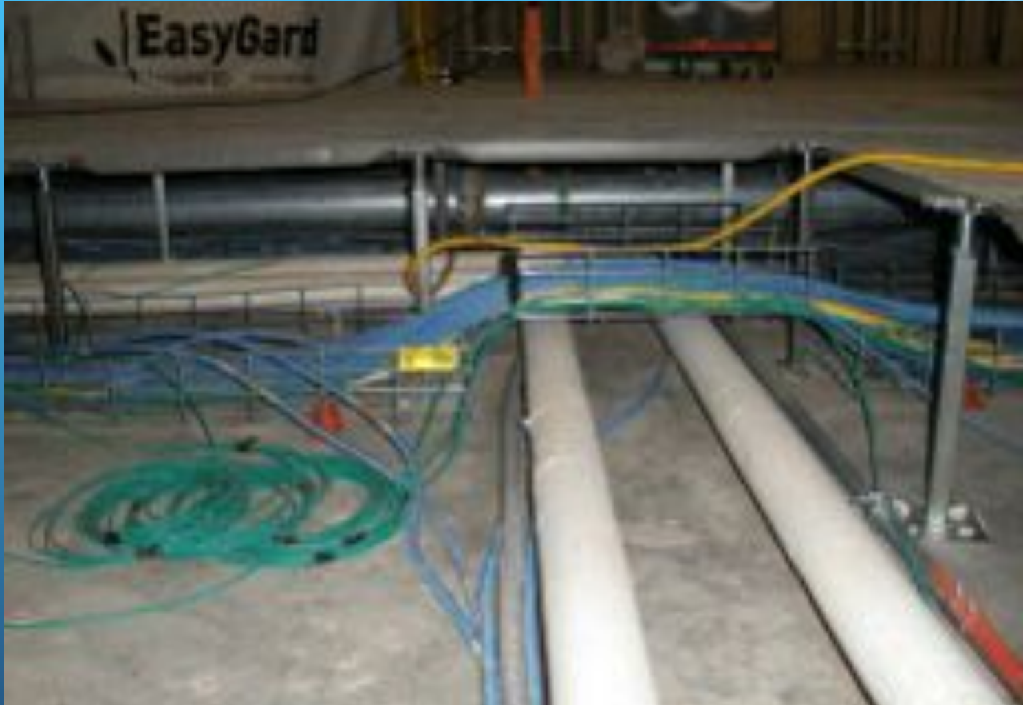
Under Floor Air Distribution System
